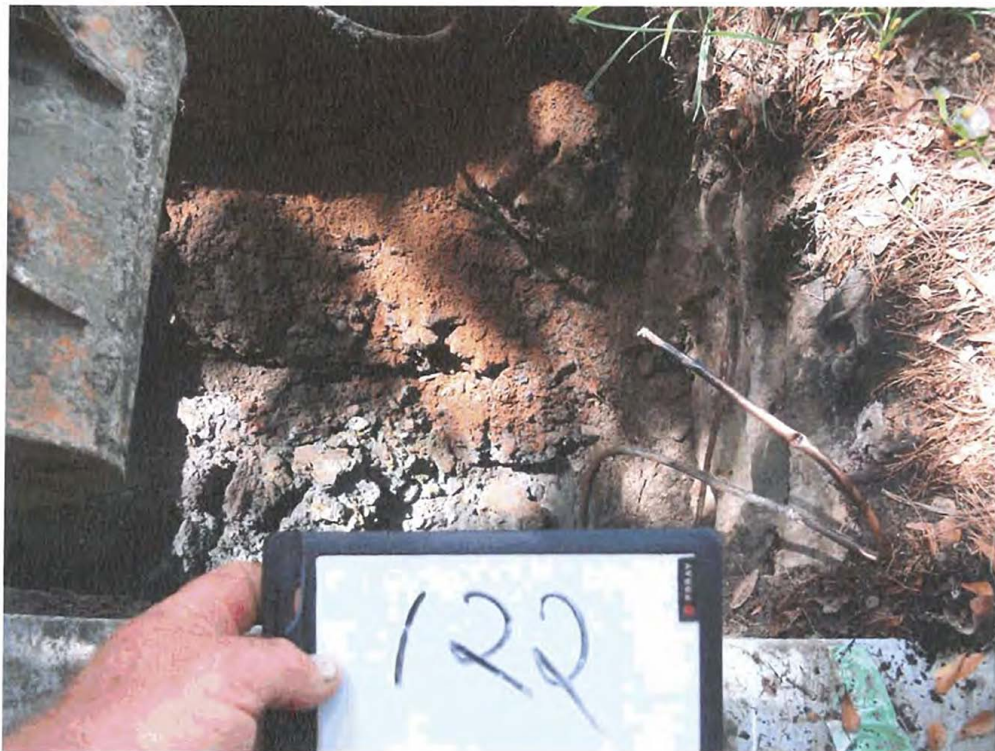
Picture 2: UST 122Banyan tank pit after removal of tank.
